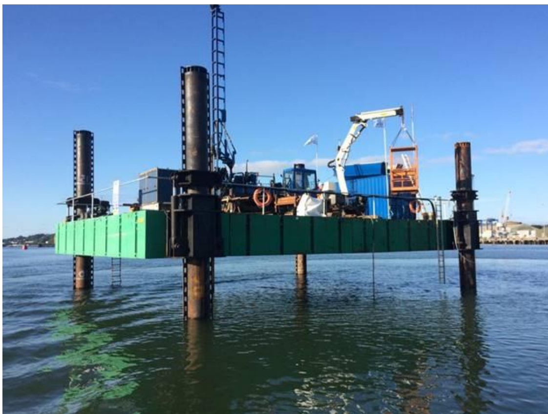
Plate 1: Photograph of the GII Jack-up Barge that facilitated the works.
